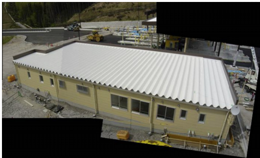
Fig. 1c. Photo of the building-B on August 26, 2007.
